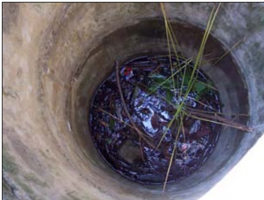
Figure 39: A well filled with garbage.
