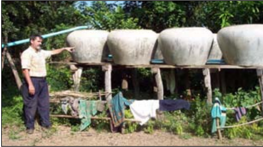
Figure 27: Small scale entrepreneurs interconnecting jars and selling water (In this case from a shallow well).
