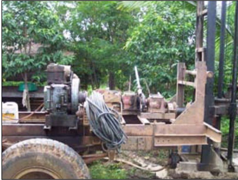
Figure 47: The drilling rig nearby the Sankai River.
