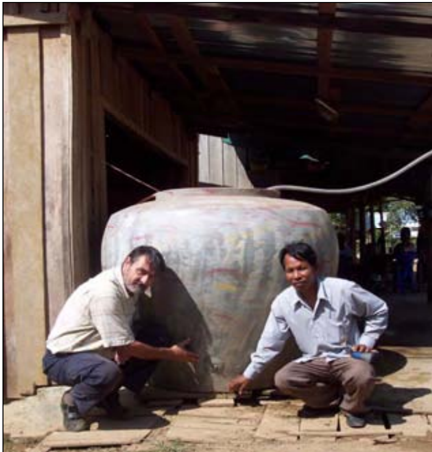
Figure 26: “Built-in “connections” at the bottom of the jars allowing for discharge and future interconnections
